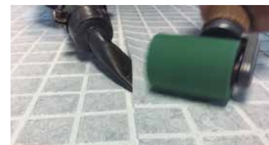
Overlap welded seams
