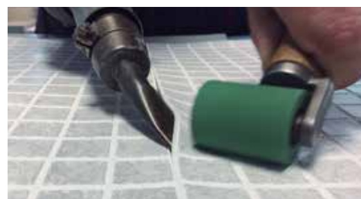
Butt welded seams
